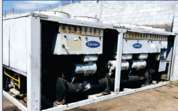
CHILLER CARRIER GRANDE PORTE 30GX (240TR) C/BOMBA
